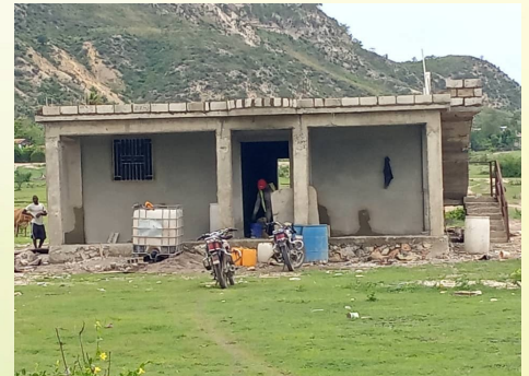
SiCC progress as of July 2024
